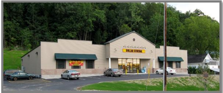
Figure 1: Use of Fenestration to break up a long expanse of blank wall.
